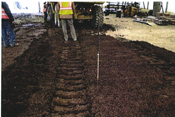
Figure 9 – North side lift 1, 12 inch loose
